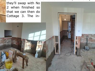
surer's have commissioned contractors to strip out the damaged plasterboard and take out the kitchens and radiators as you can see.
