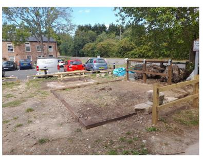
At Sandiacre Lock, we have made some progress. We've proved that no bats reside in the lock walls and we've surveyed the garden levels and the resident drains to help us to plot a course to reroute the sewer between the trees. We also have an option in principle to take a few houses off the main sewer that may work for us. We are now waiting for people to return from holiday to get a conclusion drawn and design moved on. As before we progress slowly, but surely.
