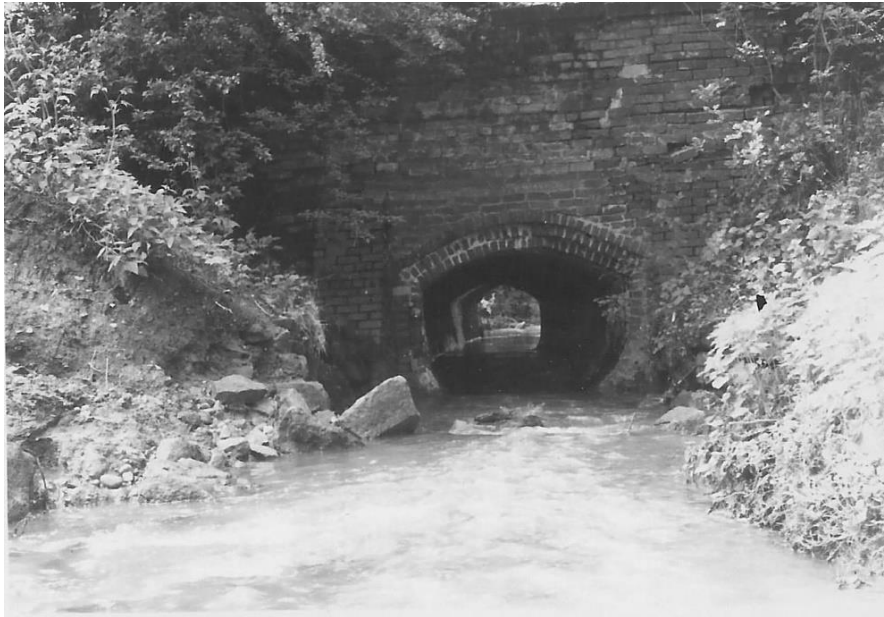
This is a picture of the culvert taking the Ock under the canal at Borrowash Bottom lock.
